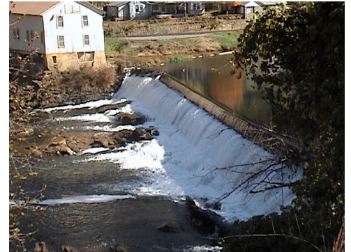
Dillsboro Dam, Tuckasegee River
