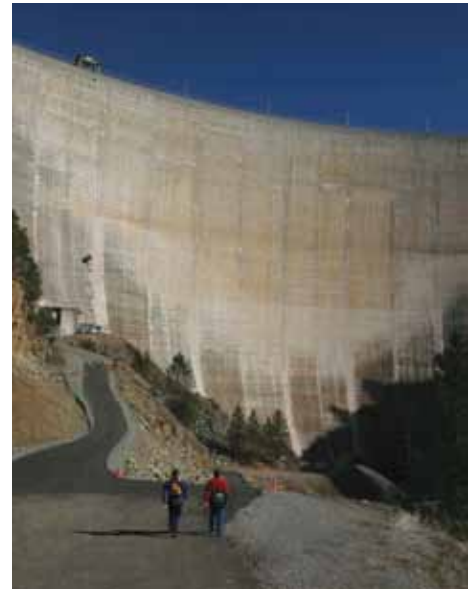
Bullard's Bar Dam on the North Yuba (CA) is part of the Yuba/Bear/Drum-Spaulding Relicensing Project.
