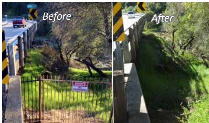
Latrobe Road Bridge on the Consumnes River (CA). Photos by Dave Steindorf
