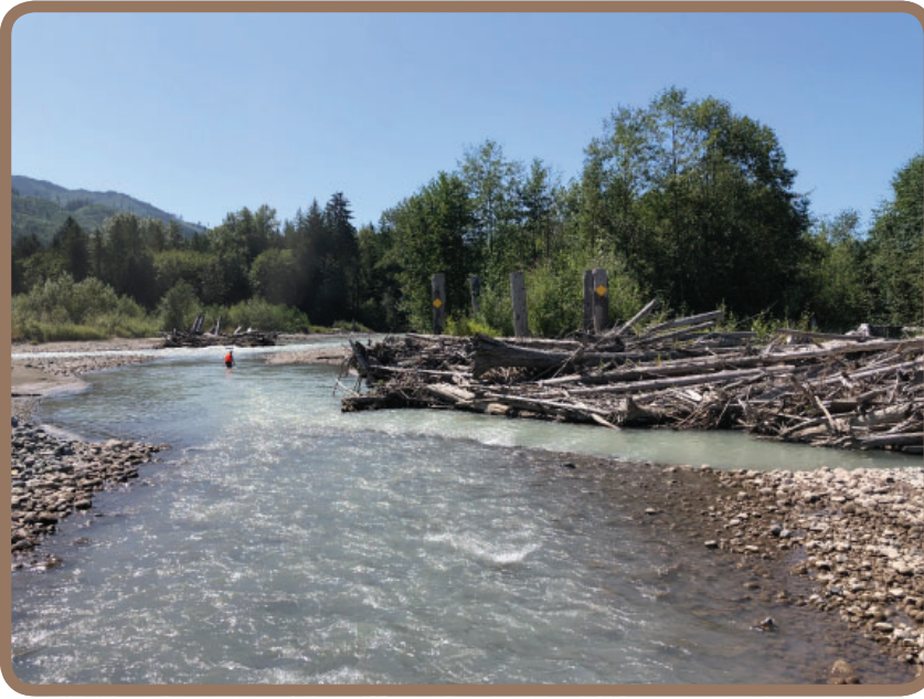
ELJ with accumulated natural wood in Farmhouse Reach. Photo credit to Lindsie Fratus-Thomas, Nooksack Indian Tribe.
