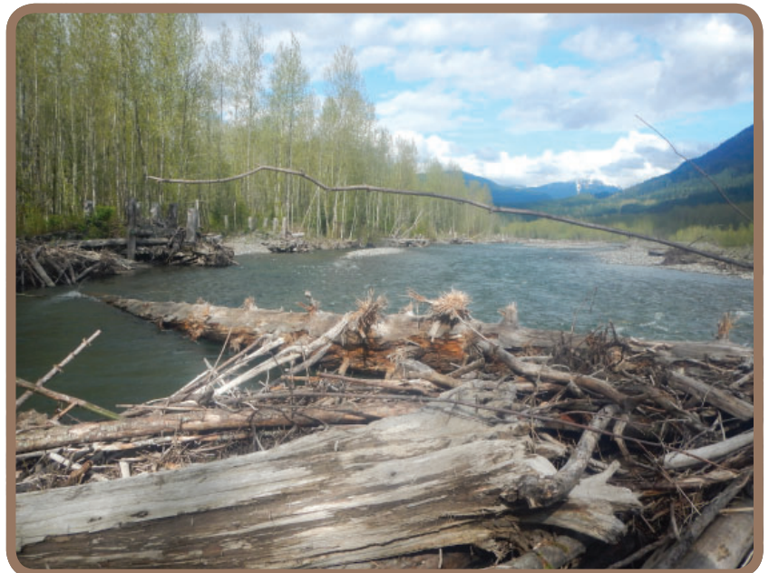
View immediately upstream from the ELJs at Farmhouse Reach. Photo credit to Lindsie Fratus-Thomas, Nooksack Indian Tribe.
