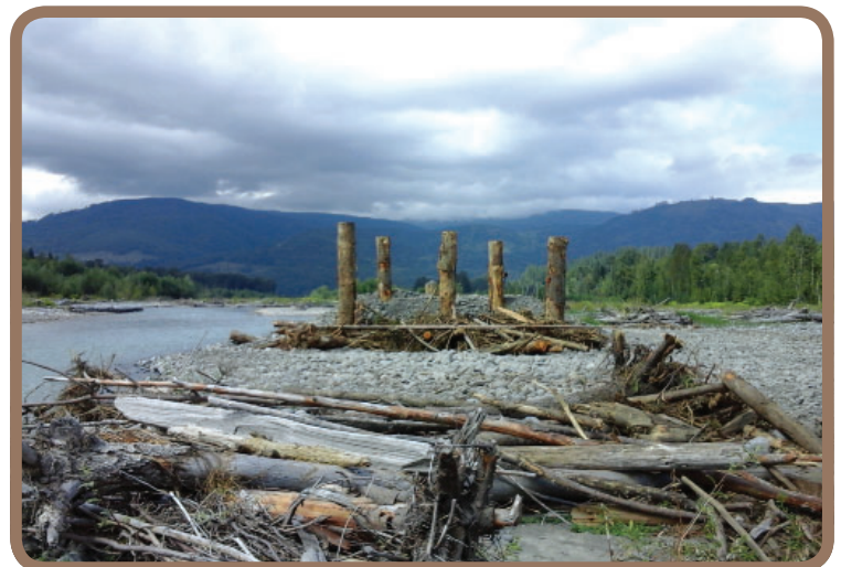
Newly constructed ELJ in Farmhouse Reach (2016). Photo credit to Lindsie Fratus-Thomas, Nooksack Indian Tribe.
