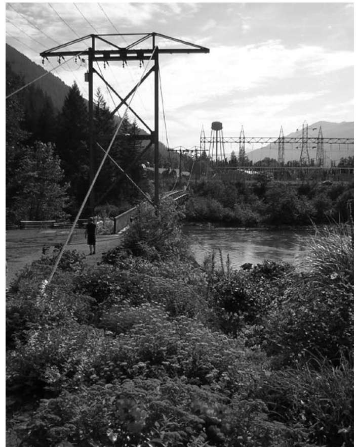
Skagit River Hydroelectric Project.
