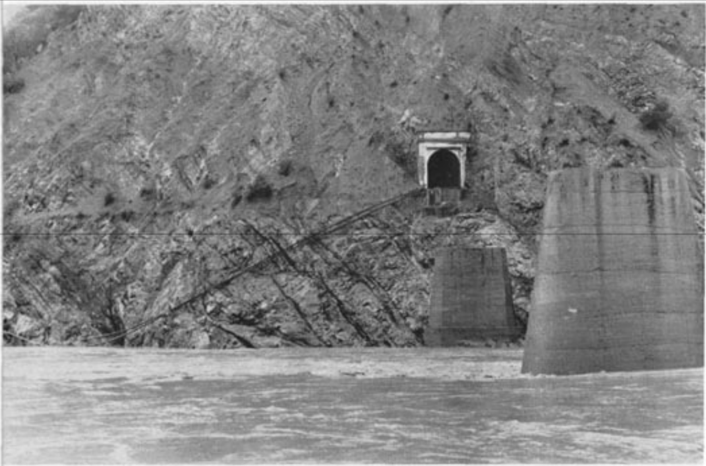
Catastrophe on the Eel: high railroad bridge washed out by December flood. Debris was deposited in the tunnel. — Photos by courtesy of Northwestern Pacific R.R.
