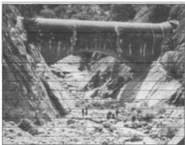
Cresta flume carrying approximately 2,000 cfs around the five mile Class IV-V Cresta run.
