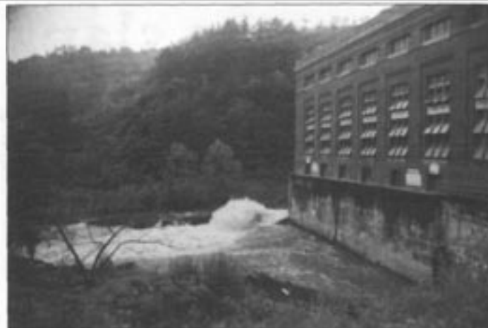
Buck Hydro tailrace on the New River
