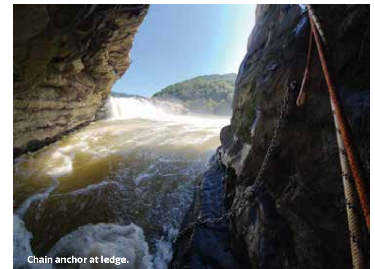
Bolt anchors above chain.
