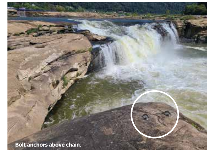
Ledge that was under the curtain.
